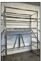
**6.** Fit 4 horizontal braces, hooks facing out using the 3T method from a seated position.
