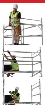
Unclip 4 x Horizontal braces from the far end of the trapdoor platform.
